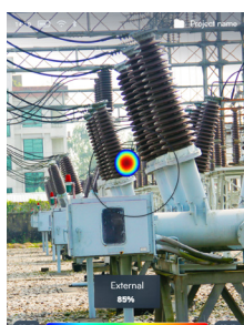
Partial discharge inspection
